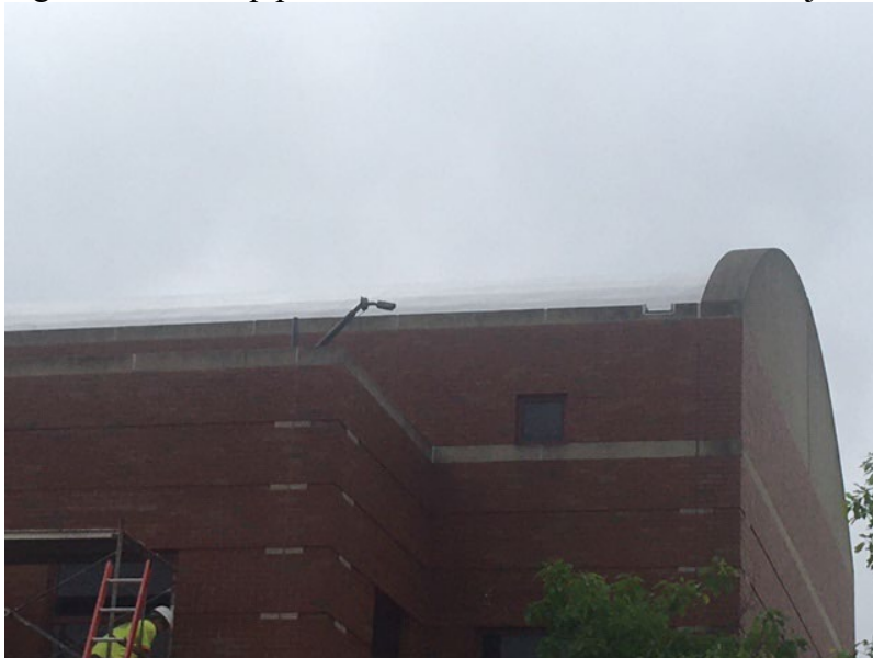
Figure 5: Close-up picture of the new PVC roof that was just installed.
