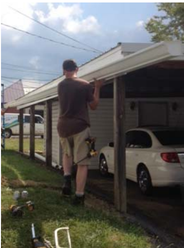
Figure 2. A construction laborer and helper assisting with an installation.
