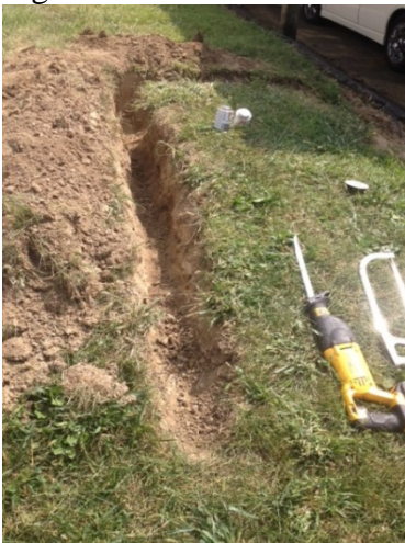
Figure 1. A trench that excavated by a construction laborer and helper.
